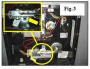
Water heater drain plug location
