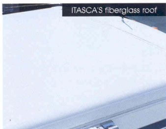
ITASCA'S fiberglass roof
