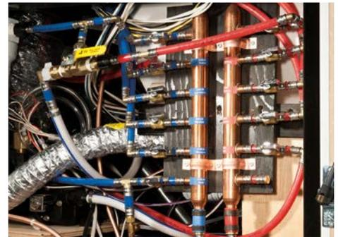
A copper water manifold comes standard, ensuring equal water pressure throughout your home. And each water line is clearly labeled and has its own shut-off valve, allowing you to isolate a single line without shutting off water to the rest of your home.
