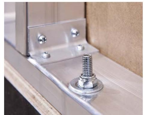
Residentially-hung sidewalls are carriage-bolted into the floor for solid construction and superior strength.
