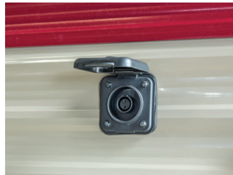
Solar Prep and Wiring
