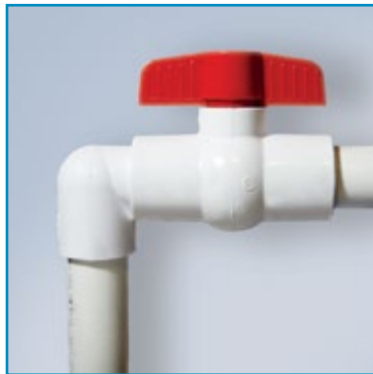
1" Fresh Water Tank Drain
