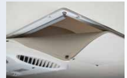
Insulated hatch covers add an additional layer of insulation to vents and sky lights.
