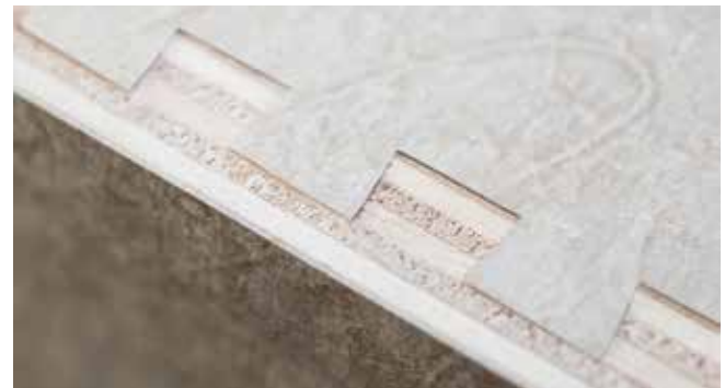
Residential dovetail drawer construction
