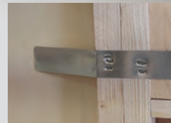
Hurricane Straps Add Strength and Safety
