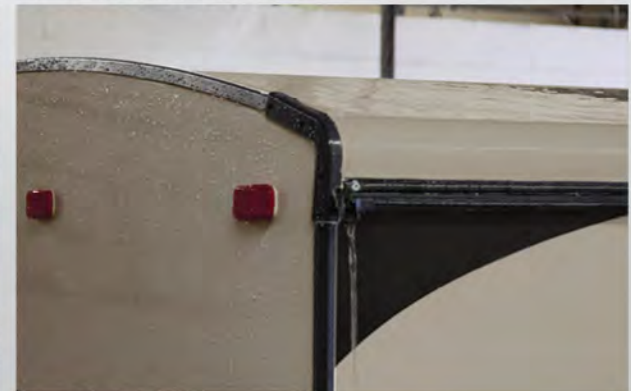
TPO Roll Over Roof
