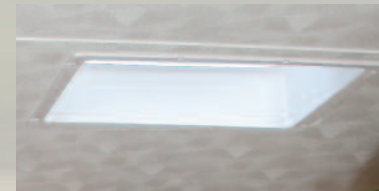
Bath skylight for natural light
