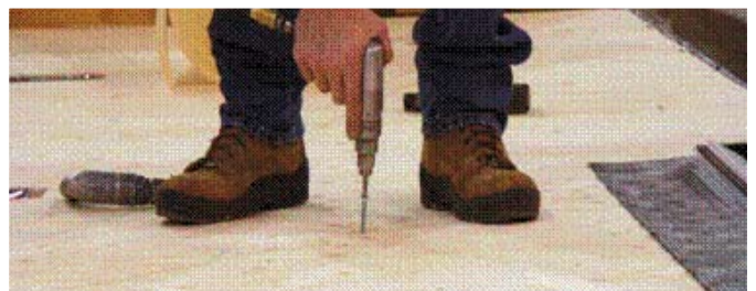
5/8" TONGUE AND GROOVE, MARINE GRADE PLYWOOD FLOOR
