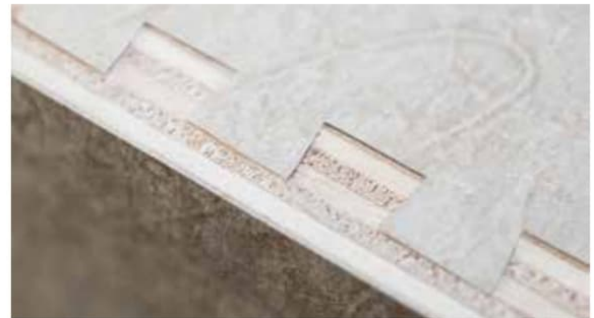
Residential dovetail drawer construction
