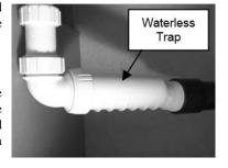
mechanical cleanout tool is used to open the drain pipe, it is important that the dry valve be removed before passing the cleanout tool through the piping. Passing a mechanical cleanout tool through the waterless valve may cause damage to the internal seal that may potentially allow sewer gases to escape into the RV interior. The waterless trap can be unscrewed from the water lines. A label has been placed near the location of the waste valve that reads as follows:
