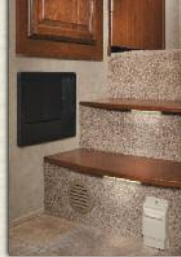
Cherry hardwood hallway steps include a central vacuum. Most heat ducts are off the floor, out of traffic areas.
