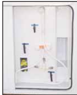
Water utility compartment with exterior shower
