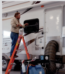
Seal Tech Air Pressure Test
