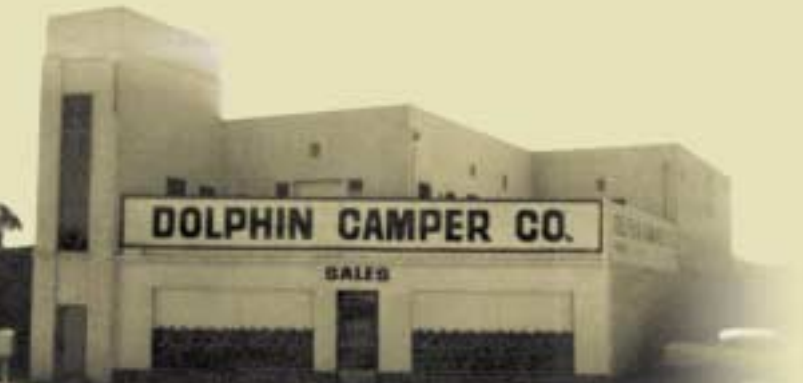
SAN FERNANDO, CA HOME OF DOLPHIN CAMPER COMPANY, PREDECESSOR TO NATIONAL RV, c.1966
