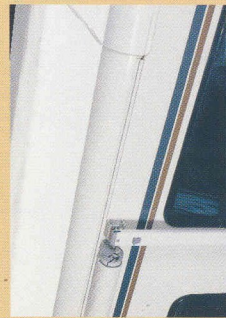
1-YEAR OLD ITASCA FIBERGLASS ROOF
