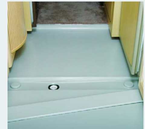
A removable cover reveals a trough with a drain that spans the lowered floor and prevents water from leaving the shower area.
