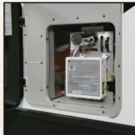
TANKLESS WATER HEATER
