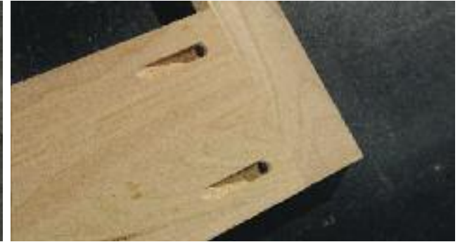
Pocket screws for structural integrity
