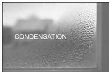
Condensation on a window is an indication of too much humidity.
