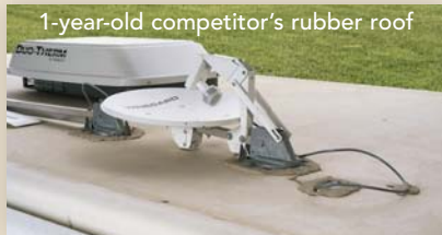
1-year-old Itasca fiberglass roof
