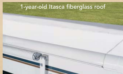
1-year-old Itasca fiberglass roof
