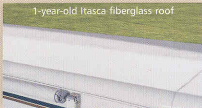
1-year-old Itasca fiberglass roof
