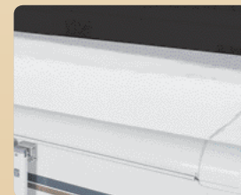
1-year-old Itasca fiberglass roof
