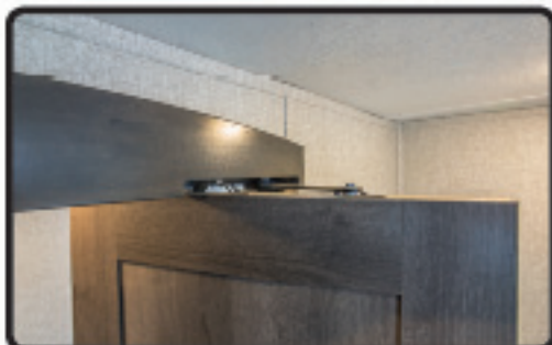
PIVOT HINGE BATHROOM DOOR ALLOWING PASSAGE WHILE DOOR IS OPEN
