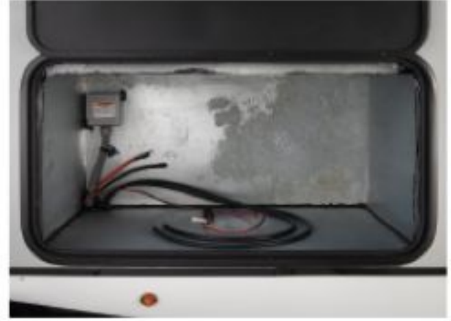
Generator Prep (Standard 27KB, 29SS)
