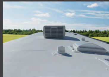
Seamless Roofing Membrane with Heat Reflectivity
