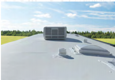
Seamless Roofing Membrane with Heat Reflectivity
