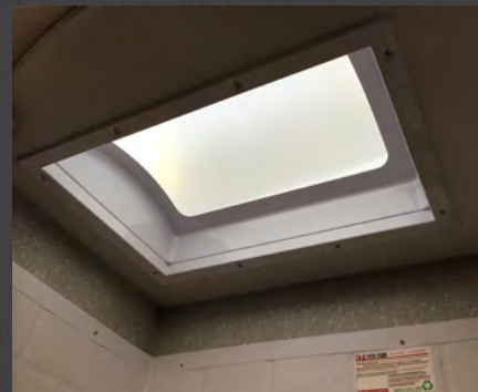
Skylight over Shower
