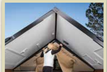
SET UP THE SIDEWALLS
