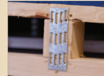
US Vertical wood studs for added support.
