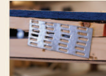
US We use large oversized nail plates on both sides.
