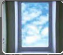
Skylight Above Tub/Shower
