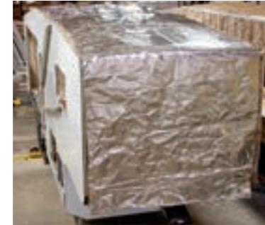
Radiant shield Therma-foil – R-38
