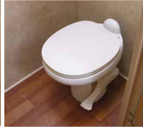
Foot flush toilet
