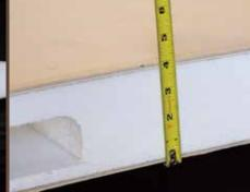
4" thick roof with built in insulated A/C ducts
