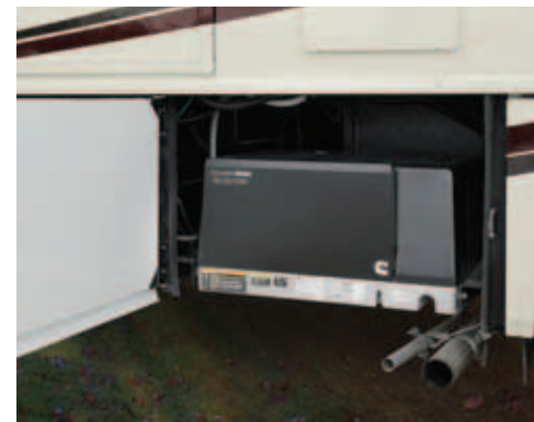
Exterior generator compartment, shown with optional Onan generator.
