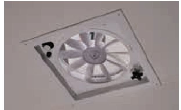
This Fantastic vent fan with a motorized lid is controlled from a convenient wall panel.
