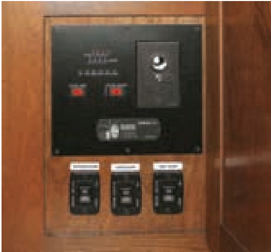
This control panel is conveniently located near the entry, hidden behind a raised panel door. Controls: (3) slide out rooms, 1,000 watt inverter, (2) power awnings, monitor panel (LP, fresh, grey & black), water pump, water heater and TV booster.
