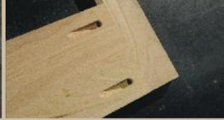
Pocket screws for structural integrity
