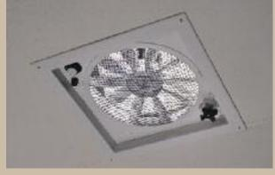
This Fantastic vent fan with a motorized lid is controlled from a convenient wall panel.
