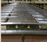
Walkable steel truss roof system
