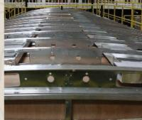
Walkable steel truss roof system
