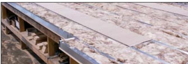
High density wool insulation blankets the underbelly frame spaces and the flooring assembly, to provide added protection for the water systems. Perimeter heating features 6" ducts and custom plenum with 5-duct heating.
