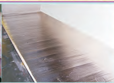
R-15 Astro-Foil Roof, Slide-Out Floor, Entire Underbelly, Additional Wrap Around Holding Tanks
