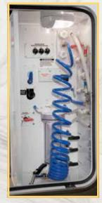
**Docking Station includes** outside shower, black tank flush, water filter, dump valves, and water tank fills for centralized convenience.
