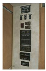
The OnePlace® Systems Center houses the PowerLine® Energy Management System (35B, 35F), which minimizes tripped campground circuits during periods of heavy usage.
