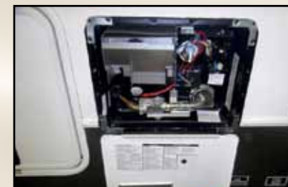
18 Gallon/Hour Quick Recovery Water Heater.
