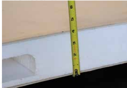
4" thick roof with built-in insulated A/C ducts.
