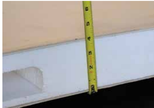
4" thick roof with built-in insulated A/C ducts.
