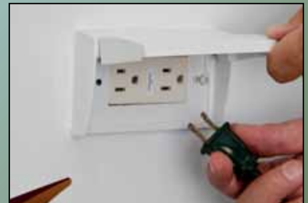
Convenient Outside GFCI Protected and Covered Outlet.
