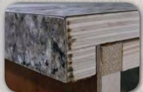
These countertops are built to last, with laminated edges and a plywood backer, instead of particle board
