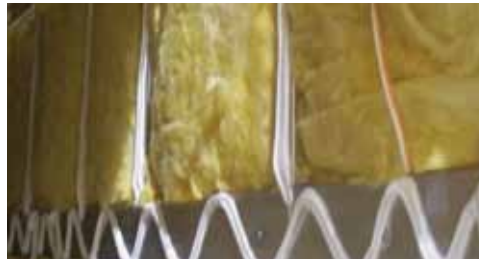
THICK SILAPRENE (475 PSI) GUARANTEES SOLID CONTACT BETWEEN THE GELCOAT AND ALUMINUM FRAME WITHOUT LAMINATION
