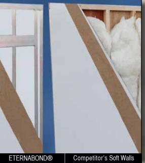
ETERNABOND® is the superior construction standard on LaCrosse. EVERY wall and main floor is bonded together to create the lightest, yet strongest construction available on any RV in the industry.
